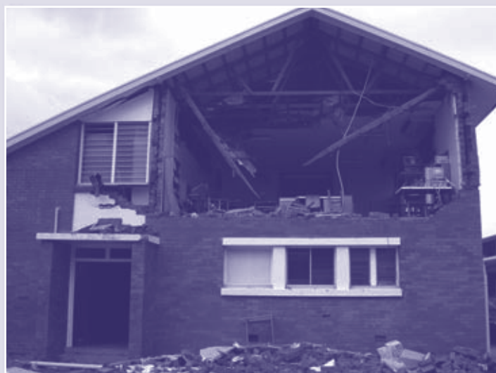
Above: The end of B Block - last classroom beside Home Economics and LOTE staffroom.
